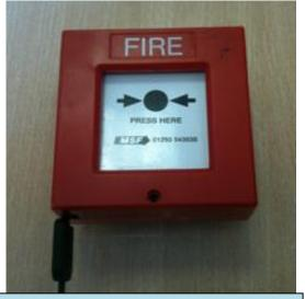
With key still in place, reattach the red cover. Use thumb and forefinger to initially screw the Allen key in.
