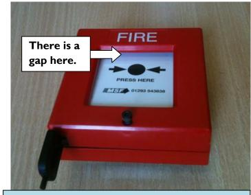
The glass will not yet be flush with the cover, there will be a gap at the top. This is normal.
