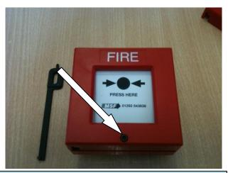
Take red plastic cover off by using top of the key (A). If stiff, use an Allen key.
