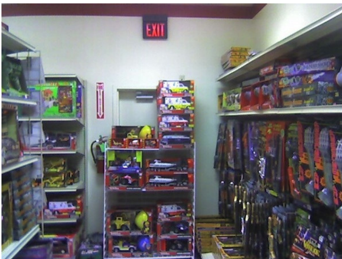
Blocked fire exit and poor access to fire extinguisher in this toy shop.
